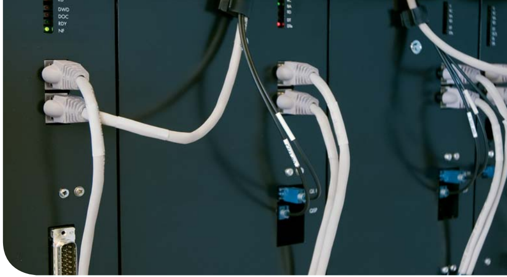
The generator for all situations
